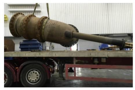
Jim continues, "The valves were isolated and the tanks drained, this enabled the team to remove the valves with the aid of a 500-tonne crane. This was a tricky process as the valves were removed through hatches within the chambers that only had millimetres of spare capacity for the valves to fit through."
